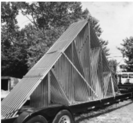
Figure 2. Prefabricated light gauge steel frame trusses were towed to the site.
