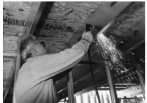
Figure 4. The Habitat for Humanity house was used to demonstrate plasma cutting of light gauge steel.
