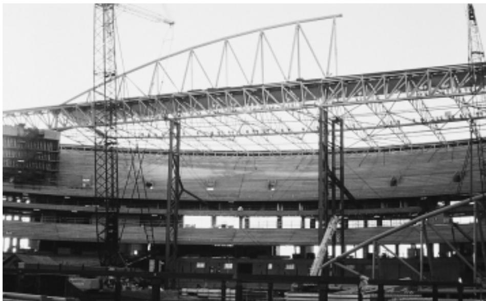
Figure 1. Installation of a section of the retractable roof.
