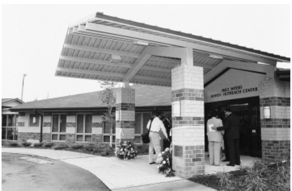
Figure 5. Cleveland's Eliza Bryant Center was framed in cold-formed steel.
