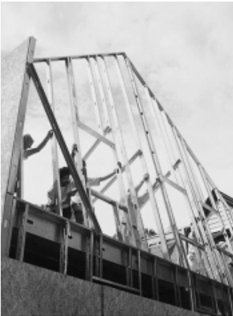
Figure 3. Volunteers installed the site-fabricated steel frame.
