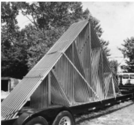
Figure 2. Prefabricated light gauge steel frame trusses were towed to the site.
