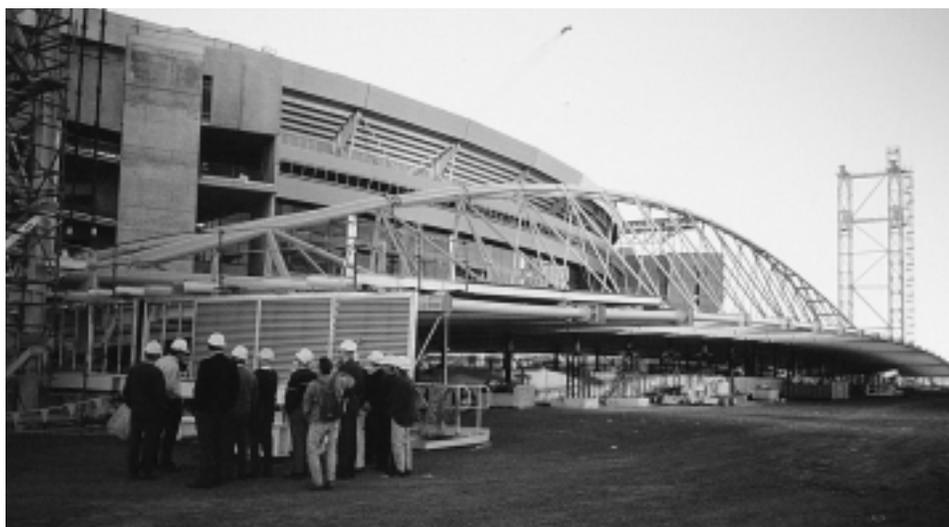
Figure 3. After field welding, a tubular truss awaits installation as part of the retractable roof assembly.
