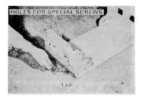
1. Run a ½" NC tap through the screw holes for strike-off plate to clean out paint and dirt. (The special screws are not locally available.)
