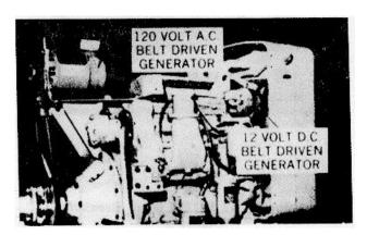
Figure 1. 12 VDC & 120 VAC Generators Detroit Diesel Engine
