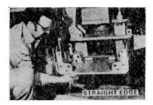
**5** Suspend screed on its safety cables. Check across the two bottom surfaces with straight edge to align flush.
