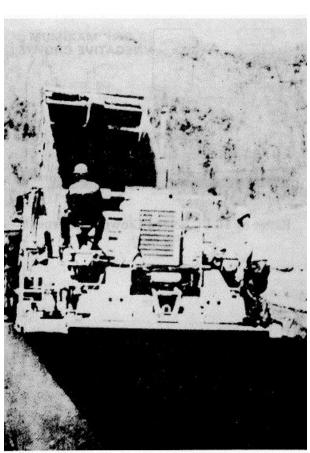
Screed Man Making Handwheel Adjustment Figure 8
