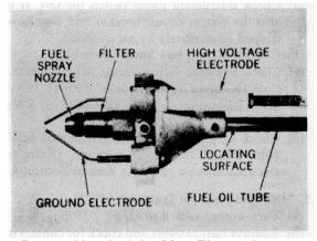
Burner Nozzle & Ignition Electrodes Figure 36
