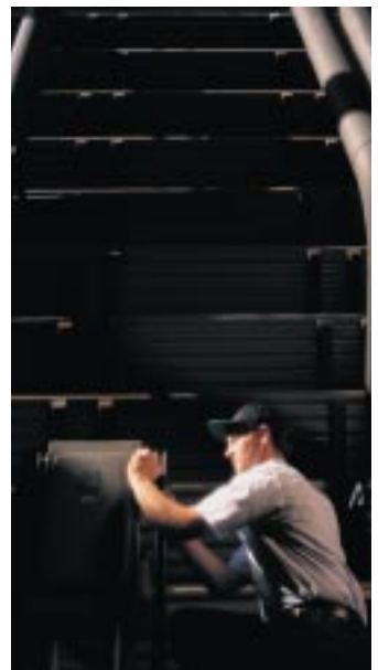
VFD control of cooling tower pumps
